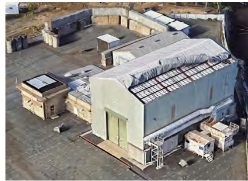
Submarine Support Facility Demolition PEARL HARBOR, HI
