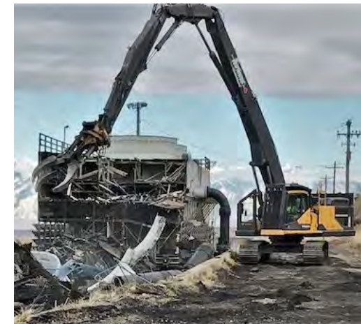
RTK Cooling Tower Decommissioning SALT LAKE CITY, UT
